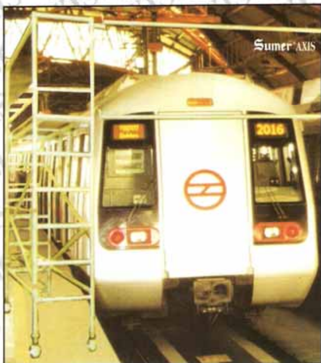
Rail - Mobile Access Platform
