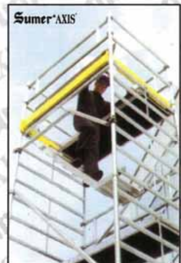
Platform Assembly, Way through Trap Door to Ladder
