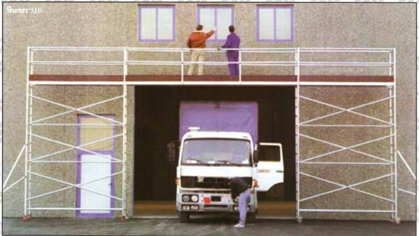
Abridge Working - Mobile Access Platform
